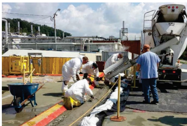
Fig. 5.43. A concrete berm being poured as part of the 3026 stabilization activities.
